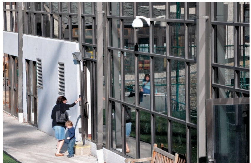
An Arecont's 180° megapixel dome camera mounted within view of one of SAR Academy's entryway/exits. The project included the installation of more than 25 new 1.3- to 5-megapixel cameras, which greatly enhance images when compared to the old analog system.
