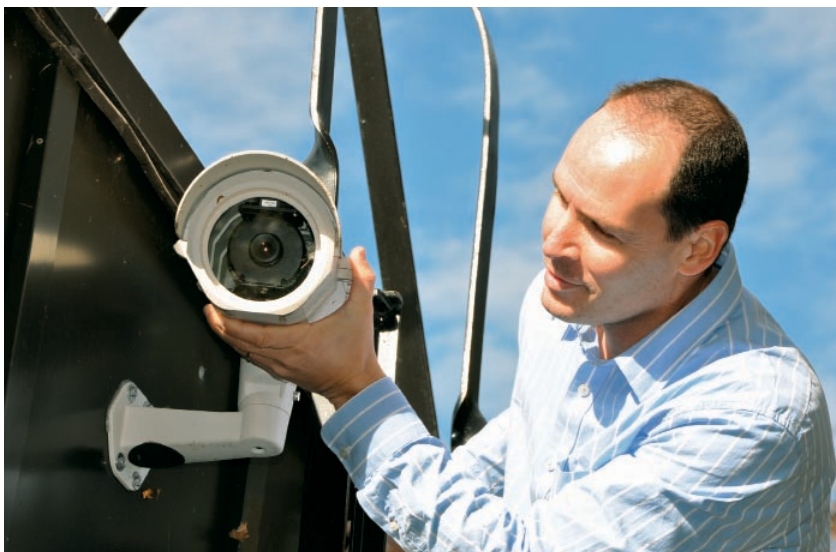
Idesco Senior Project Manager Simon Vizgan adjust the focus of one of the more than 25 Arecont megapixel cameras installed throughout SAR's campus and two main buildings. The solution helps ensure the welfare of the facility's approximately 1,300 students.
